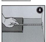
4. At the end of the first row, Put a distance of 0 mm to the wall and measure the length of the last plank to fit.
